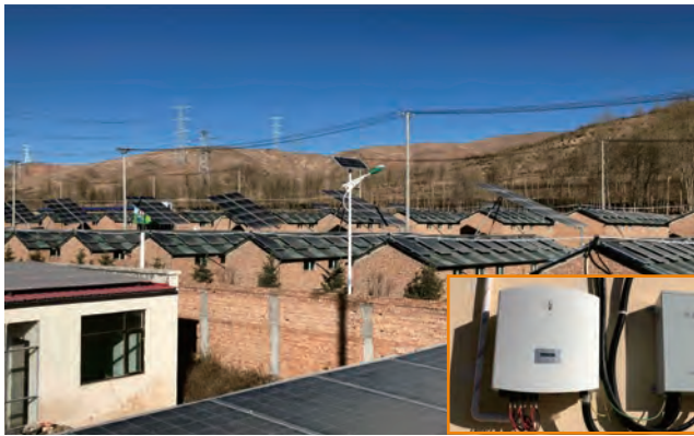
Qinghai HuzhuBanyan poverty alleviation PV Plant 2MW
