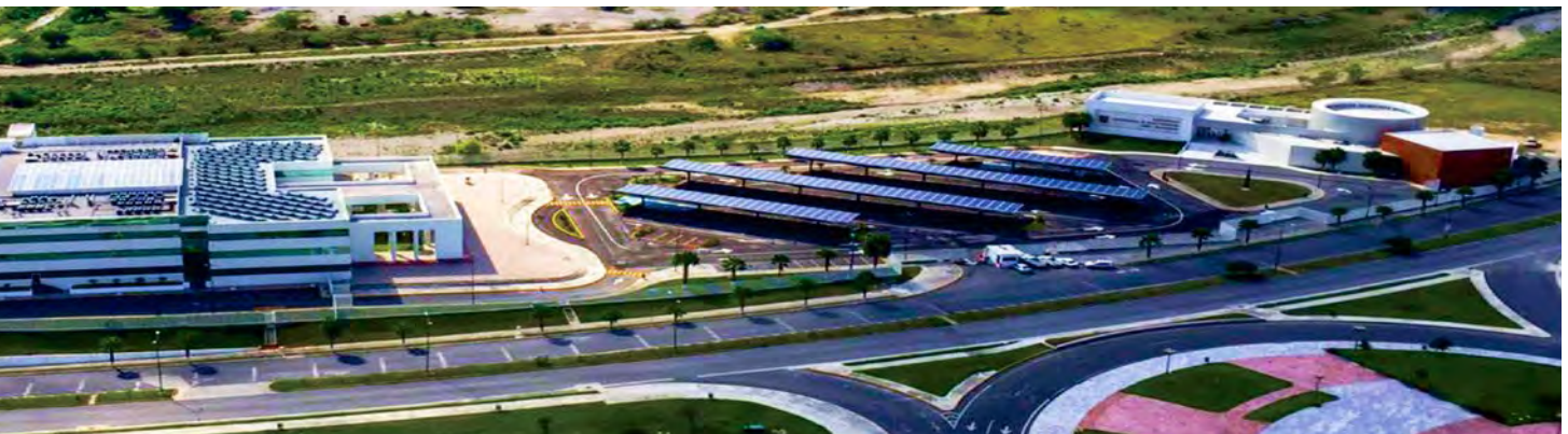
Mexico-Tamaulipas Carport, Mexico 5MW
