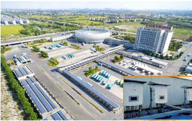
Zhejiang PINGHU Bus Station 472kW
