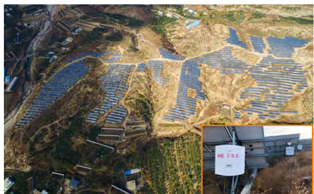
Liaoning Jiuzhai Gaizhou PV plant 20MW
