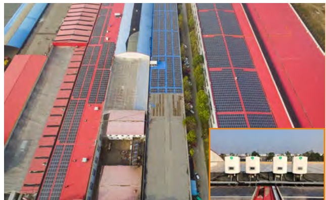
Shandong Weifang Linqupoverty alleviation PV Plant 20MW
